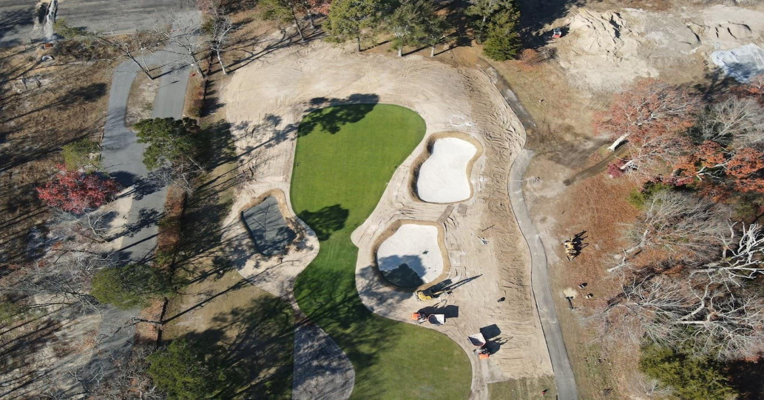
Sand install and compaction of sand on 11 greenside bunkers
