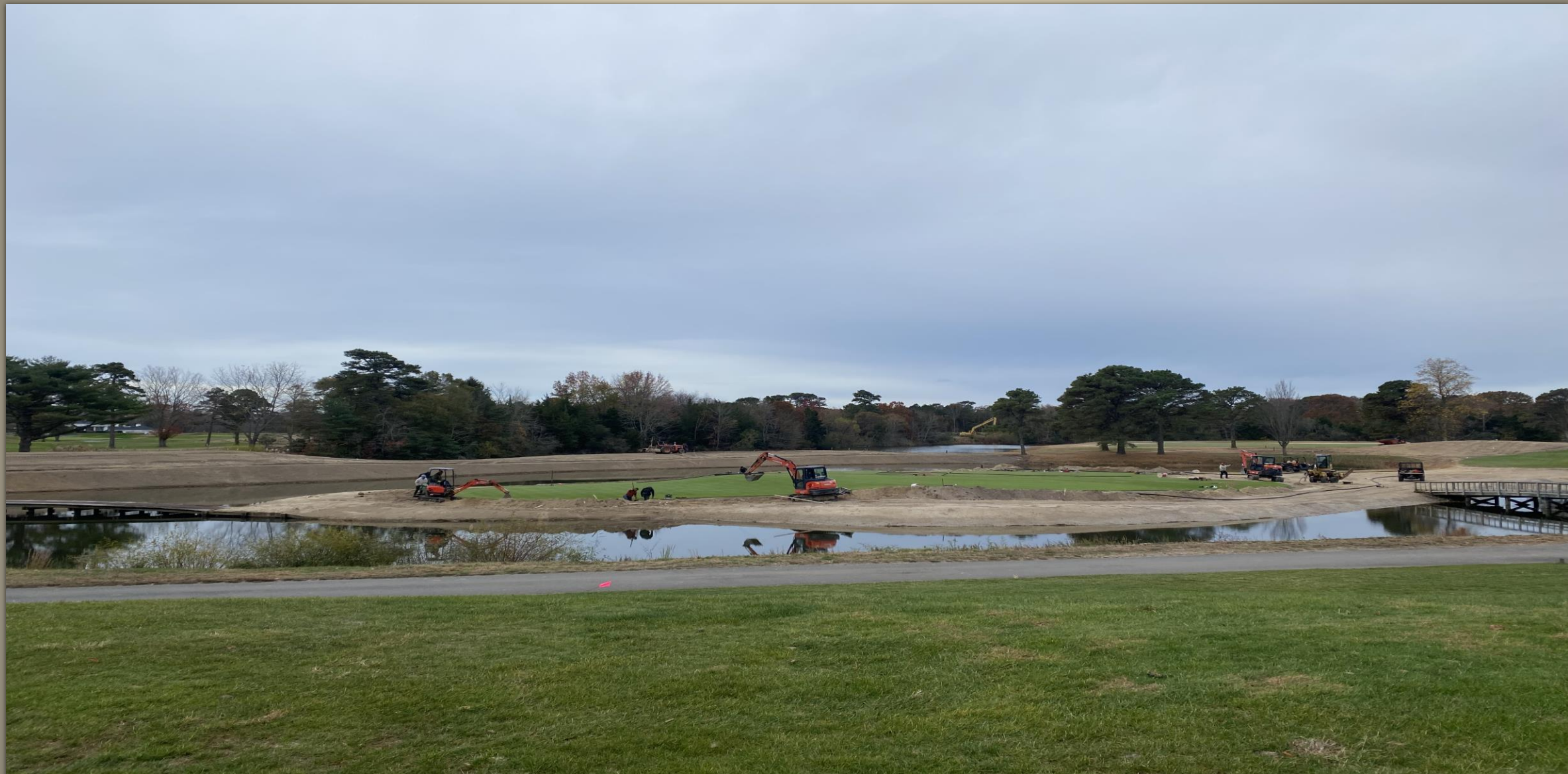
Green surround install on 15 green
