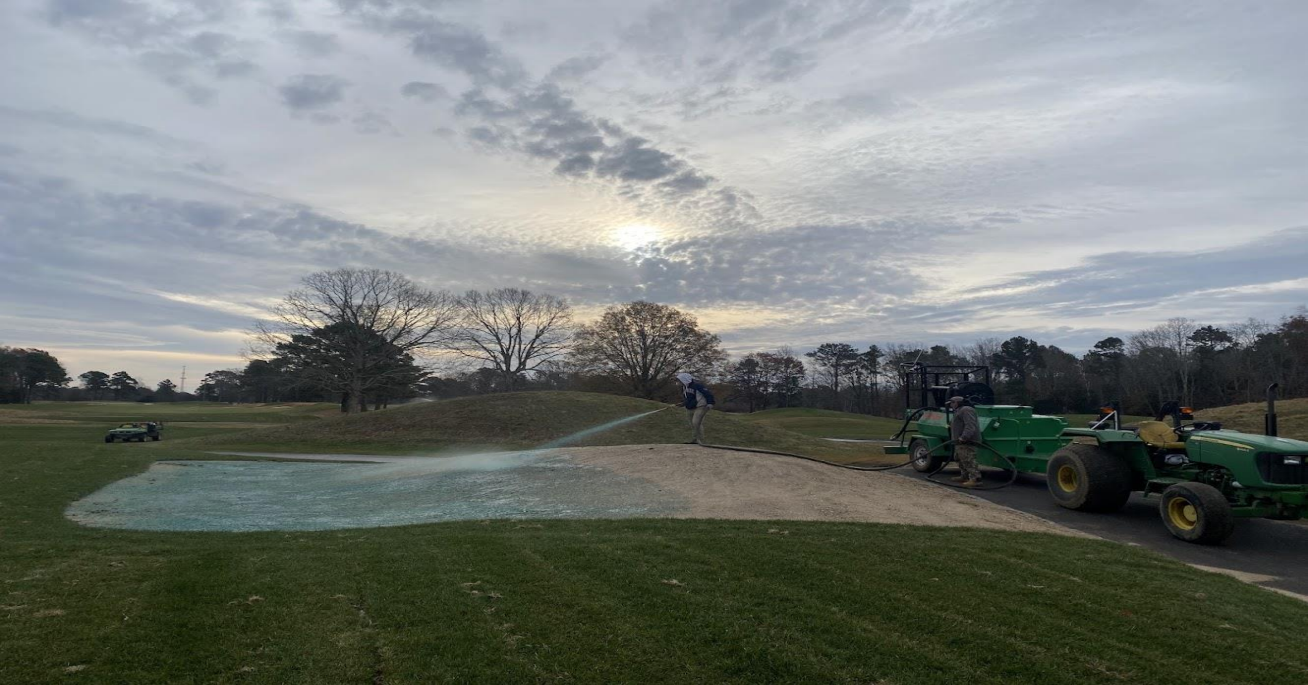
Hydroseeding 14 tee surround – blue tacking mulch used to prevent erosion and keep seed wet throughout season
